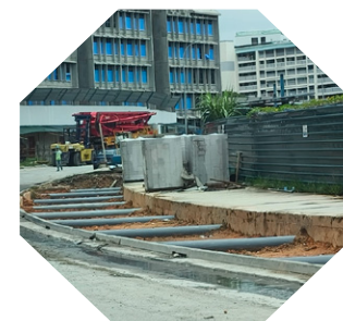
Islandwide PUB Roadside Drain Upgrading
